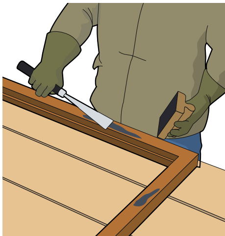
5 Rebouchage, masticage, ponçage
